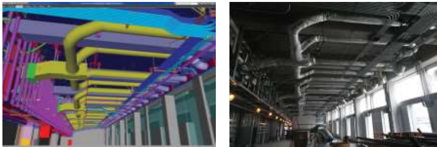
Figure 3 A model in BIM and its reality, (URL-2).
