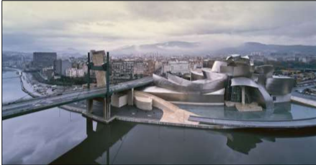
Fig. 1. Bilbao Guggenheim Museum by Frank Gehry
